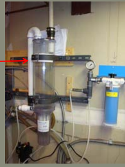
Columns are installed downstream of amalgam separator.
