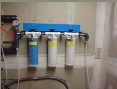
Columns are installed downstream of amalgam separator.
